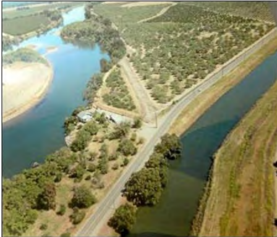
Figure 4.6-2: Aerial Photograph of “J” Levee along Sacramento River
