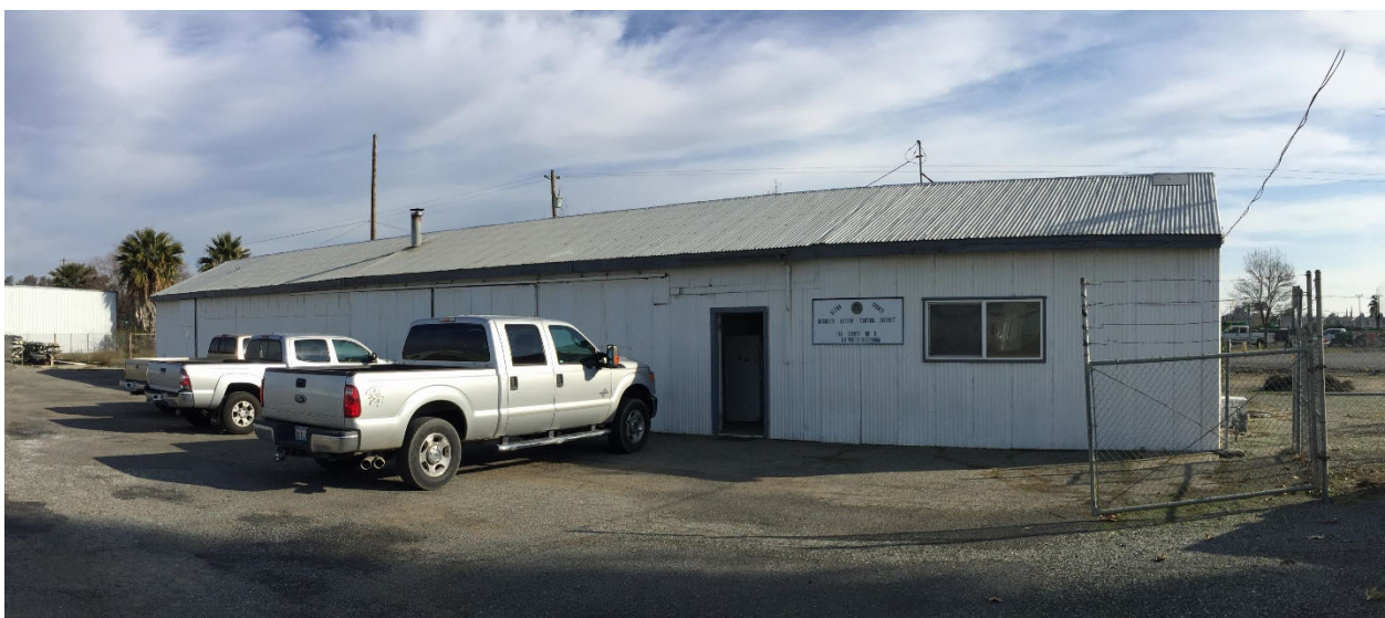
GCMVCD Building – West Side
