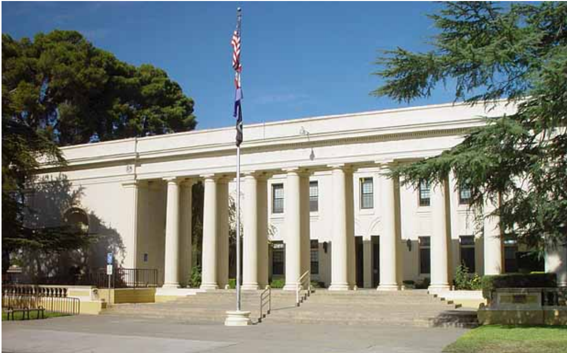
Memorial Hall Building – Willows, CA
