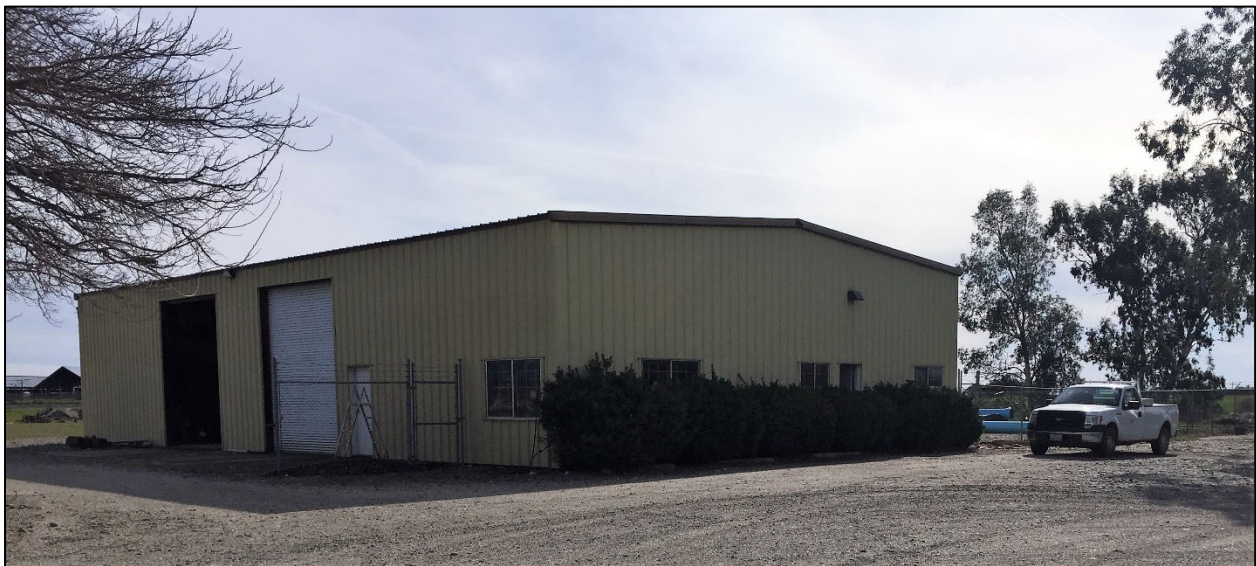
OAWD Maintenance Building
