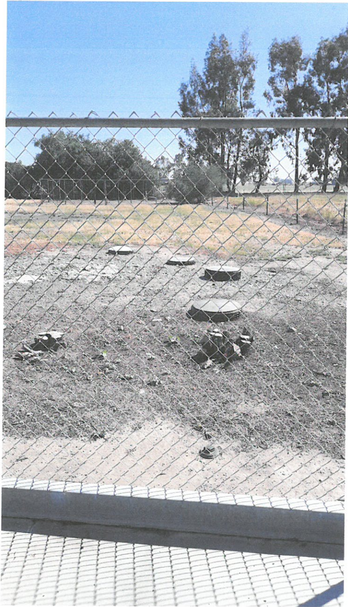
Septic tank lids as seen from building #2, on site plan page #2
