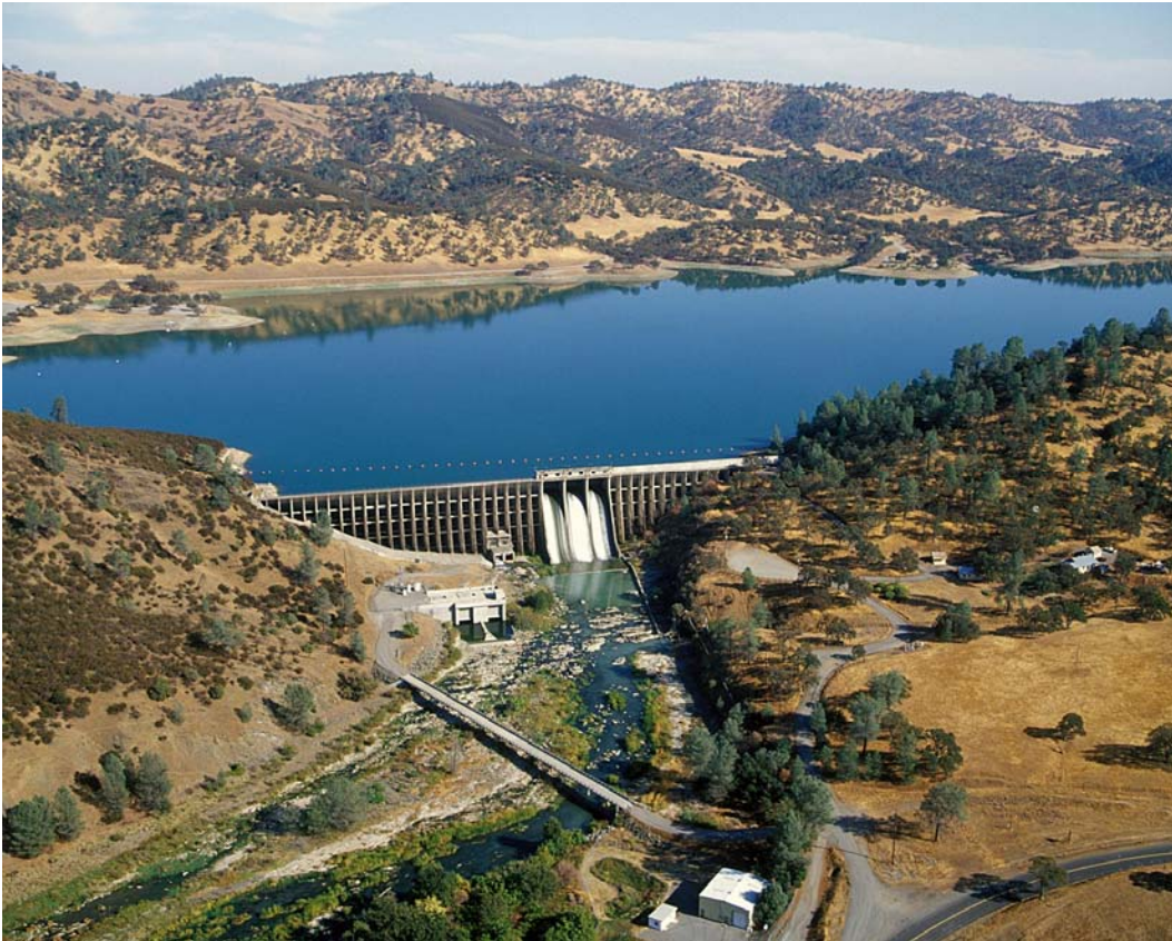
Stony Gorge Dam – Glenn County
